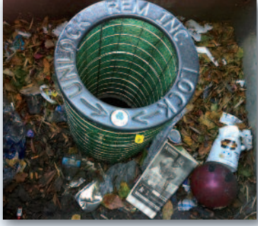
Device used to Capture Trash in Water Runoff
